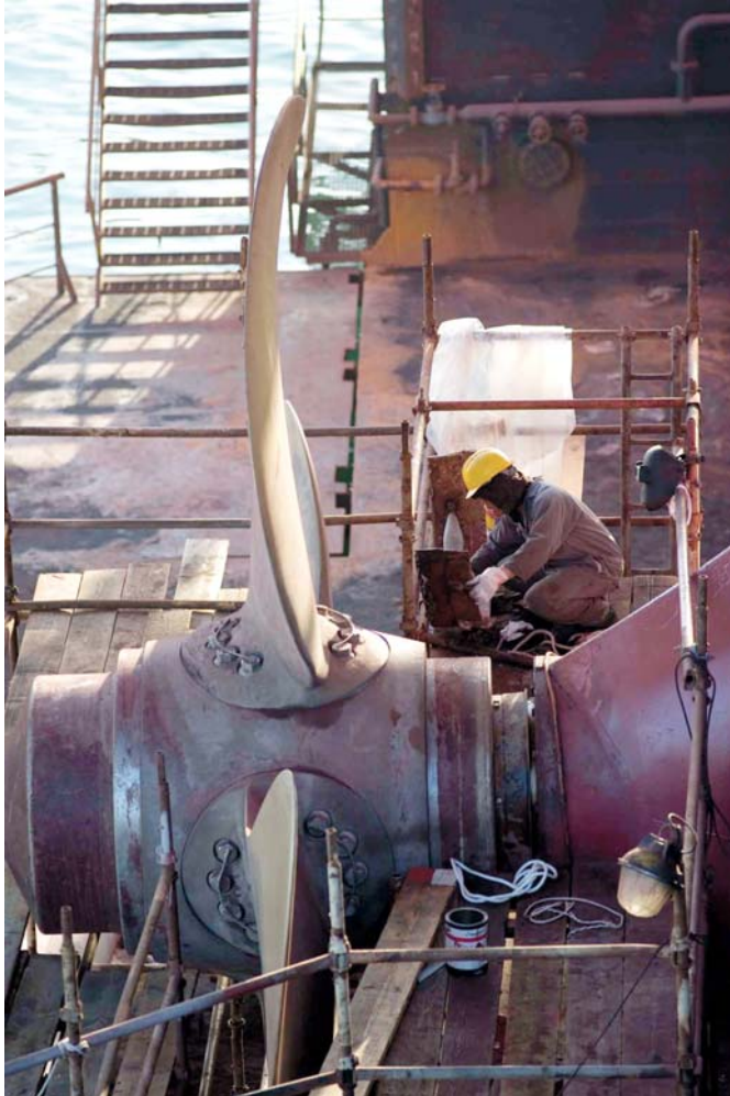
Retrofit of aft seal
